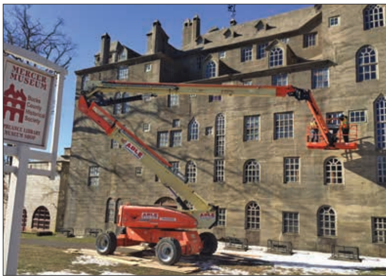
A hydraulic lift is being used to examine the condition of the Mercer Museum's windows, made of concrete.
